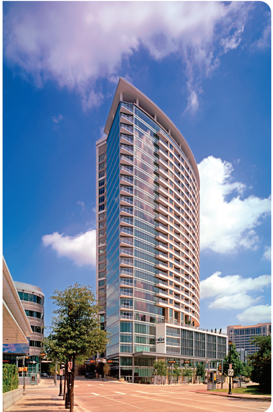
Cirque, a shimmering 28-story luxury apartment tower in Dallas, was designed with Solarban® 70 glass because of its excellent solar control performance and transparency.
